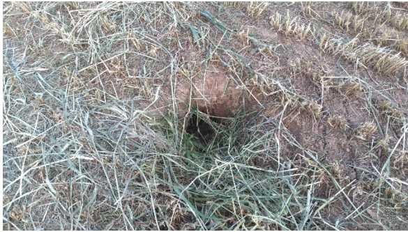
Photo – Newly developed sink hole
